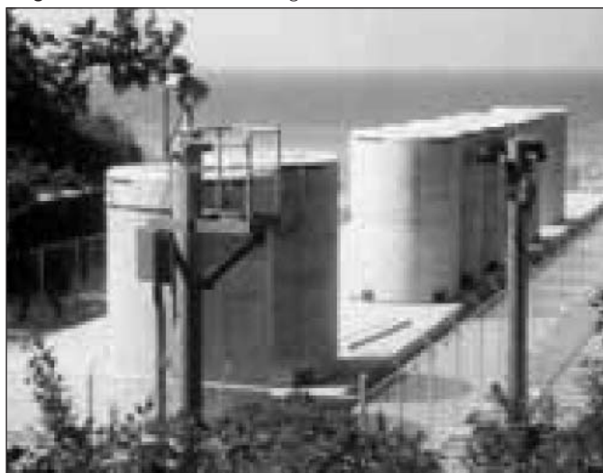
Figure 2. VSC-24 Casks in Storage
