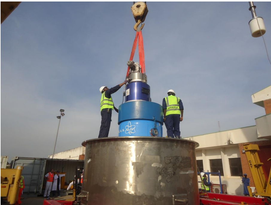
Figure 2: CERT personnel loading HEU Core into transport Cask
