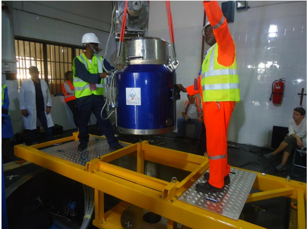
Figure 1: CERT operators discharging HEU Core from NIRR-1 Vessel
