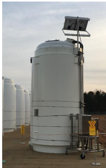
Figure 4. High Burnup Research Project Cask at North Anna ISFSI
