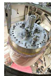
Fig.11: Cask handling preparation cell, to unloading
