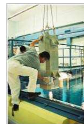
Fig.3: Transfer system for loading TN-MTR at RR site
