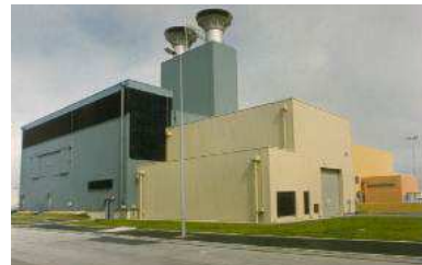
Fig.29: Outside view of La Hague EEVSE facility
