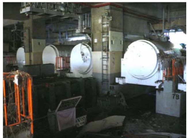
Figure 4 Cask storage facility after the Great East Japan Earthquake
