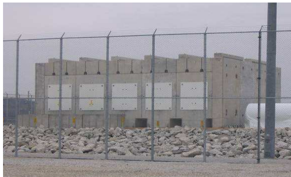
Figure1: NUHOMS ® System at Fort Calhoun storage facility, USA
