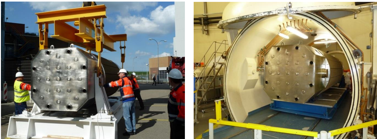
Photo 7a and 7b : handling the TN17/2 cask outside and inside Borssele NPP
