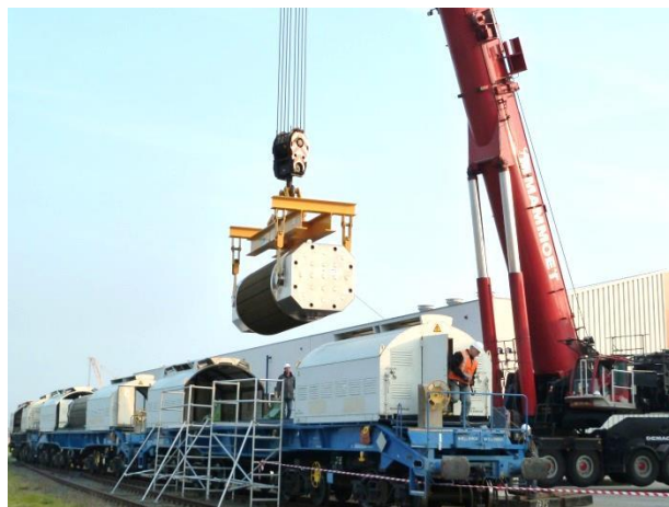
Photo 8: cask transfer at COVRA by mobile crane
