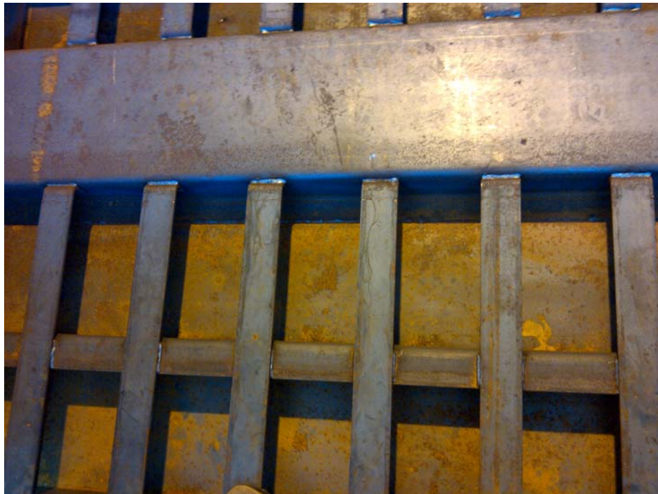
Figure 2: Exposed internal steelwork lattice of disposal container base structure
