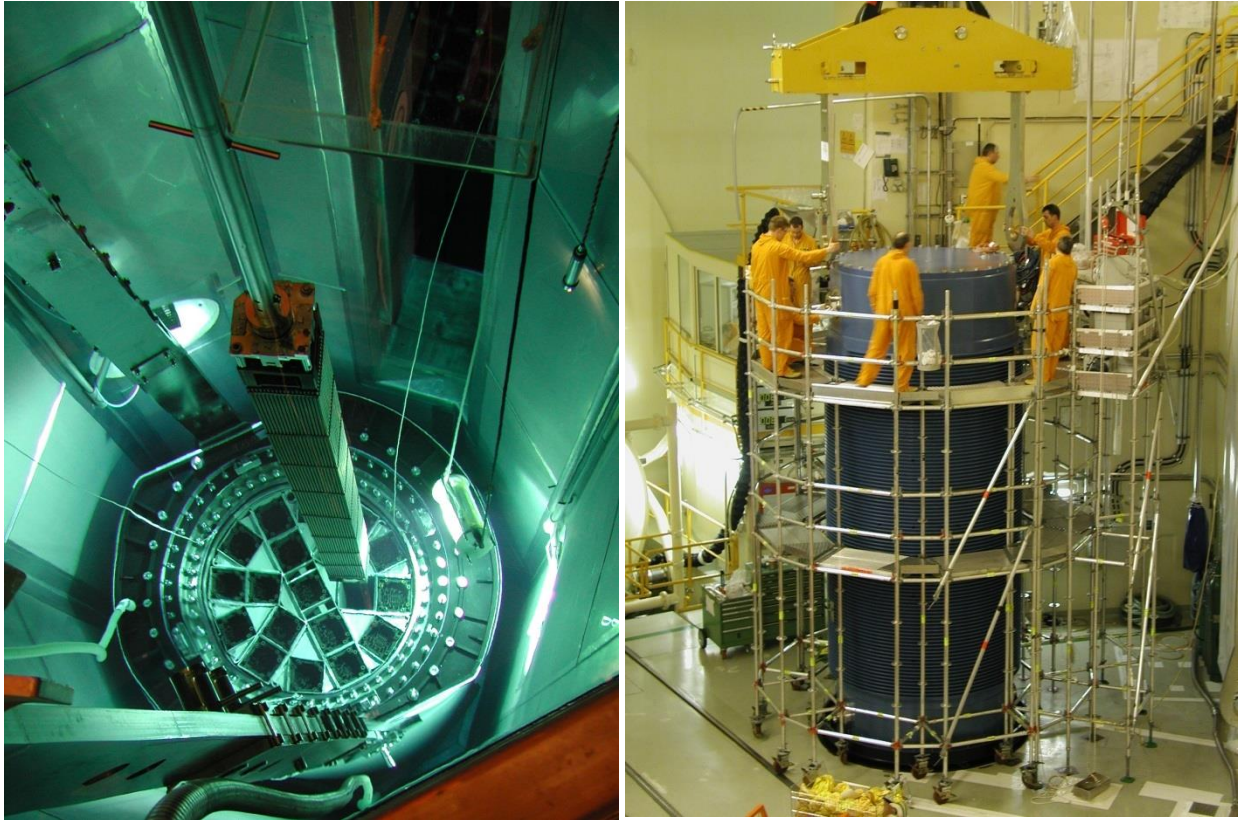
Figure 6: Cask loading and handling
