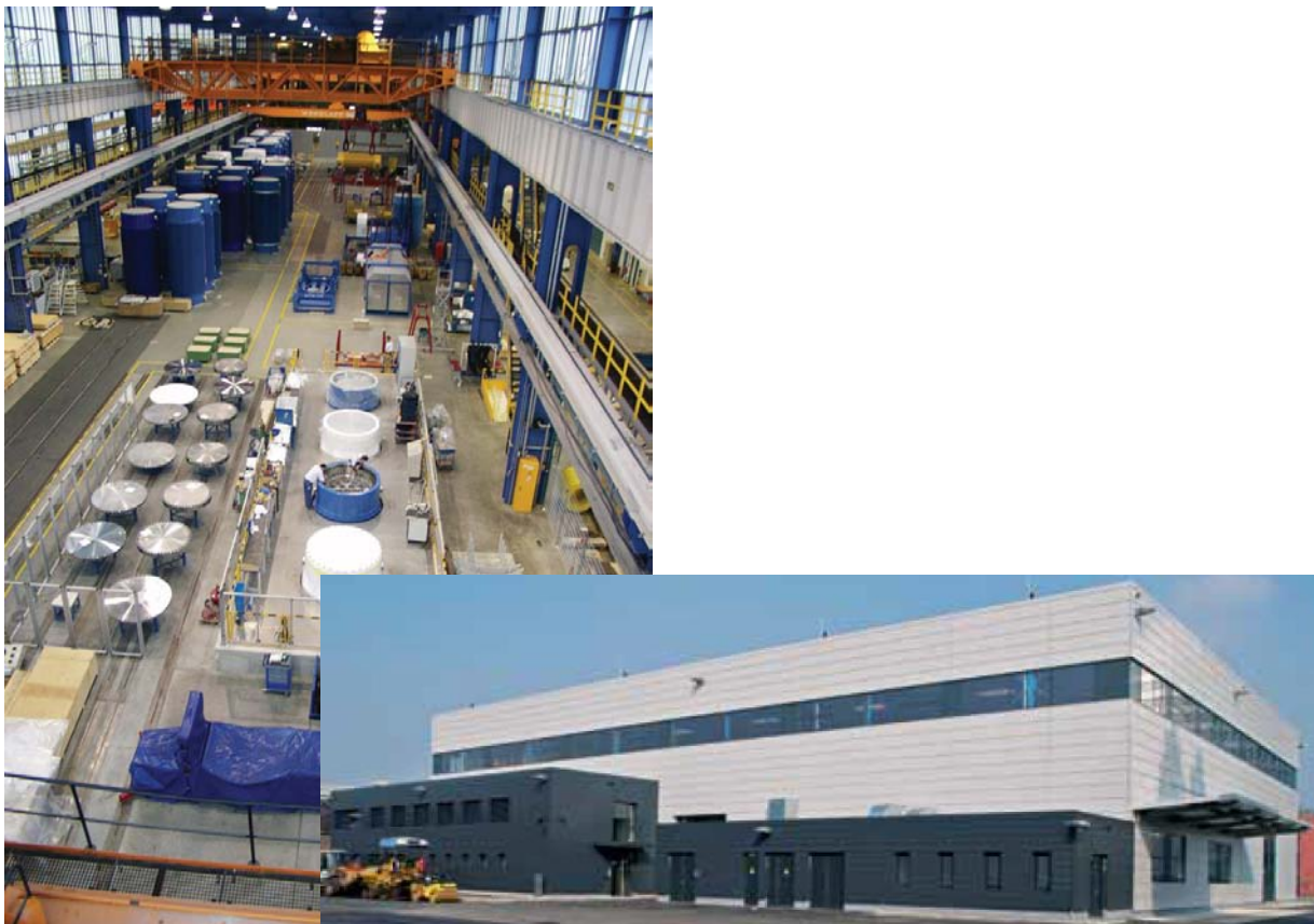
Figure 5: GNS-Manufacturing plants I and II in Mülheim / Germany
