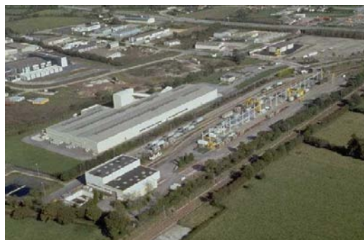
Figure 7. Railway Terminal at Valognes
