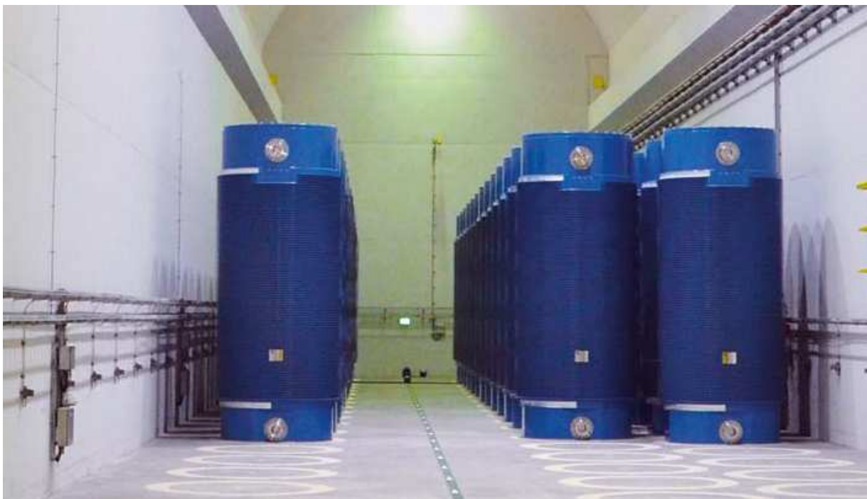
Figure 1. Example for storage of dual purpose casks in a storage facility in Germany (from BfS Jahresbericht 2012)
