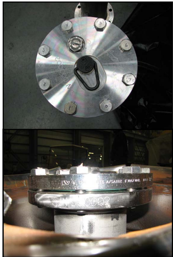
Figure 15. CCC End Drop Inspection
