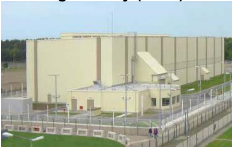
NPP Emsland cask storage facility (RWE)
