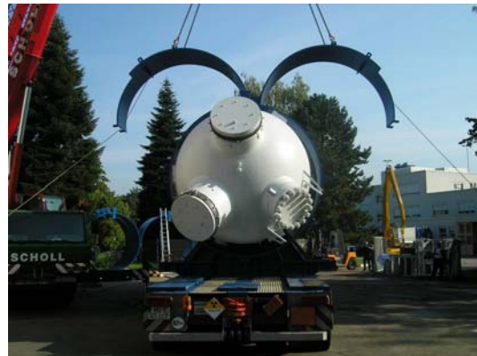
Figure 6. Assembling of shielding
