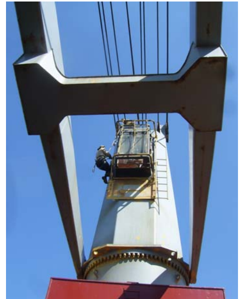
Photo 2. MCL Trader crane being cleaned and painted.
