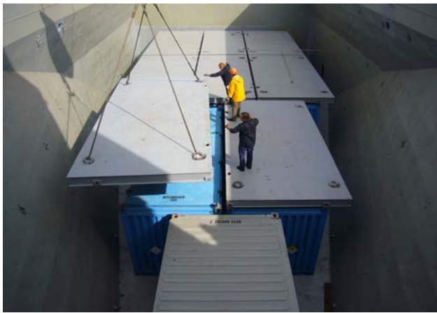
Photo 5. Special radiation and biological protection covers for the ISO containers.
