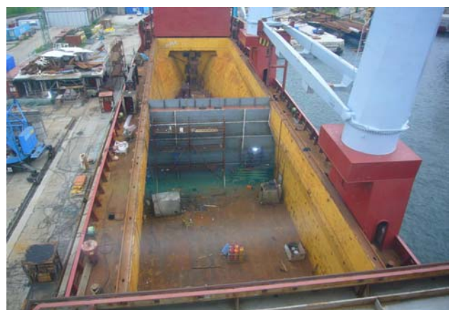
Photo 4. Bulkhead being built to separate vessel Hold No. 1 from Hold No. 2.
