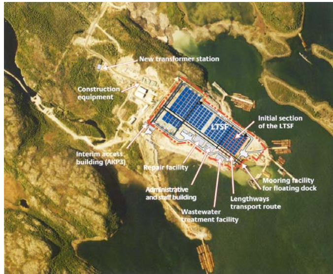
Fig. 1: Construction area for building the LTFSF
