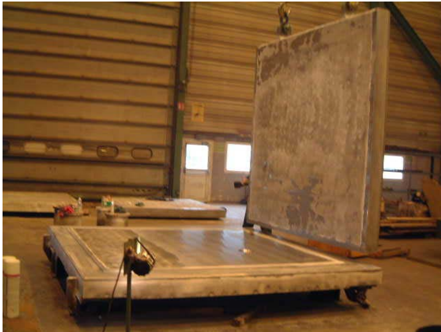
Picture n°4 = set up of the first forged wall
