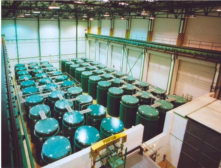
Figure 2. Photograph of the completely loaded ISFSF Dukovany I
