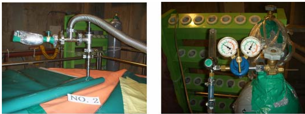
Figure 6. Leakage Inspection of the Cask.
