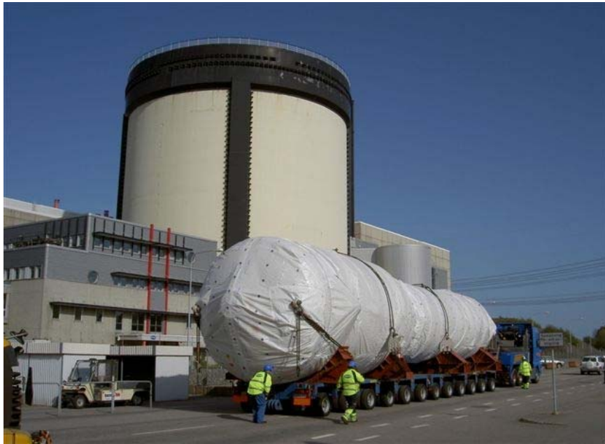
Figure 2. Steam generator leaving Ringhals NPP, Sweden
