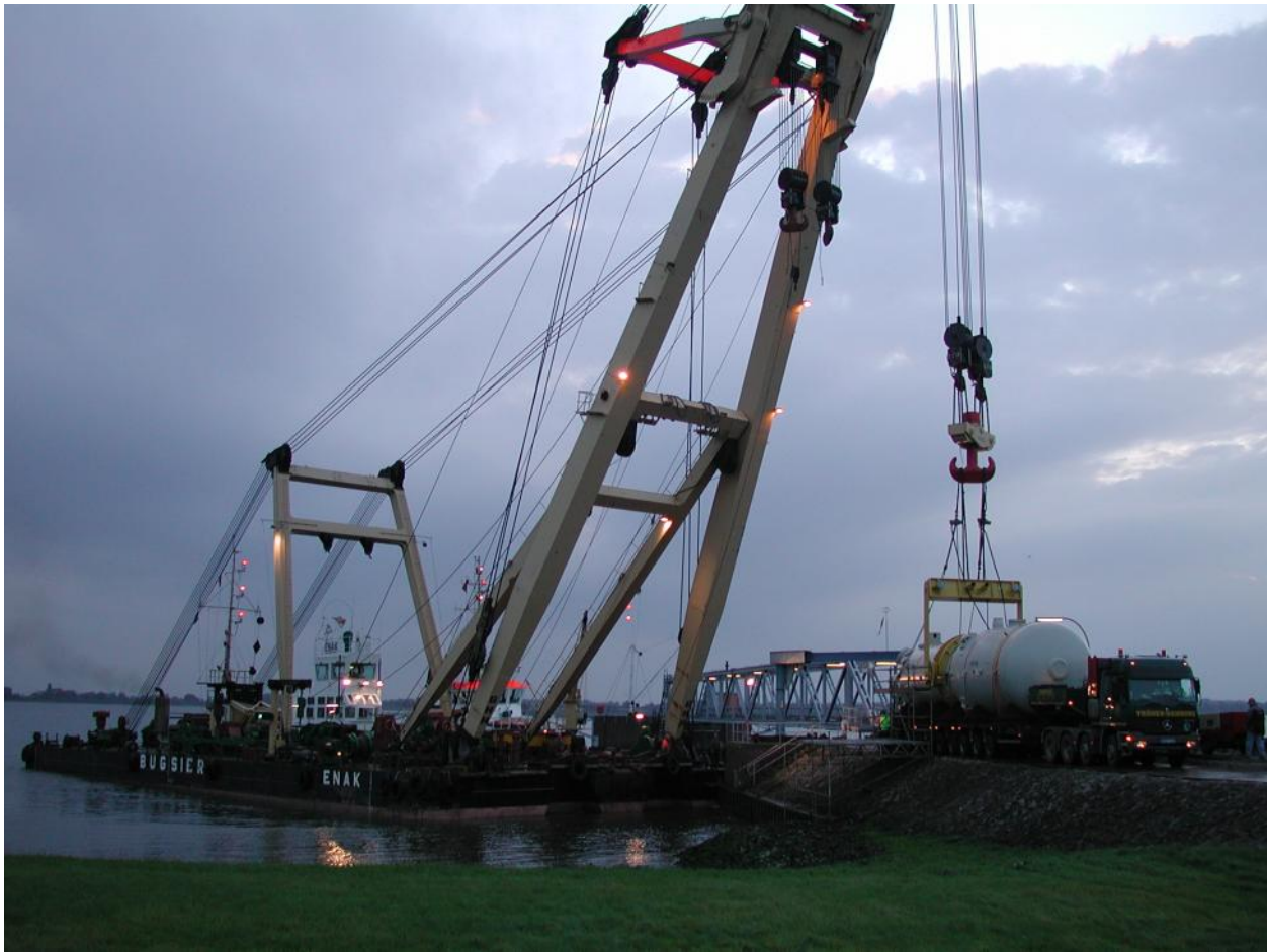
Figure 5. Transfer of the steam generators by floating crane
