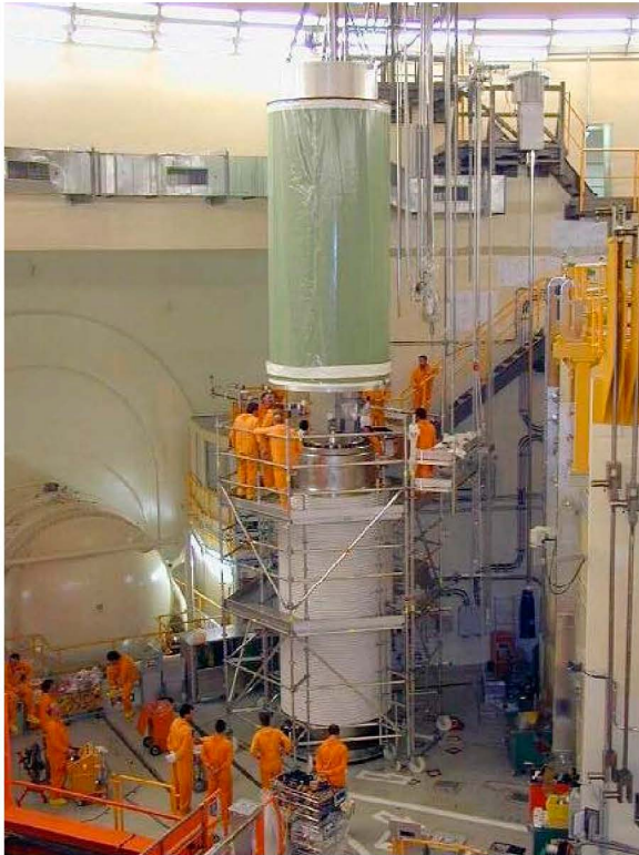
Figure 5 Plastic skirt prepared for fitting to transport flask
