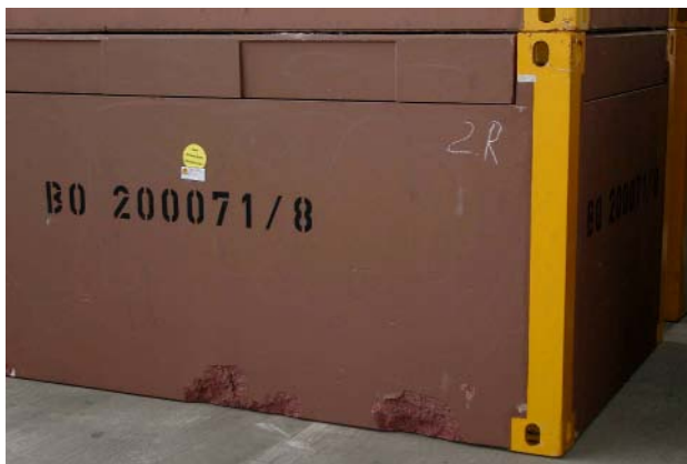
Fig. 2: Spalling on the lower edges of a concrete container
