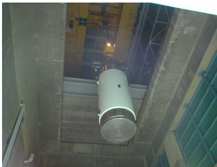
Fig. 9 Cask carrying-in to the fuel building
