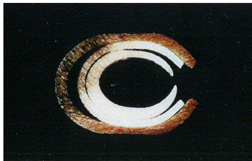
Photo. 1 Gasket section after long-term heating (120°C)
