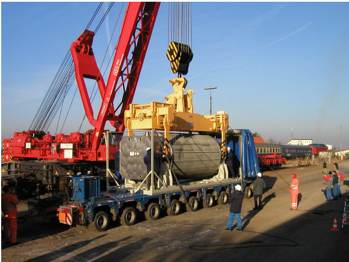
Fig. 1: TN 13/2 flask from KKG Grafenrheinfeld is being transferred from road trailer onto railway wagon by means of a railway crane at Gochsheim train station.
