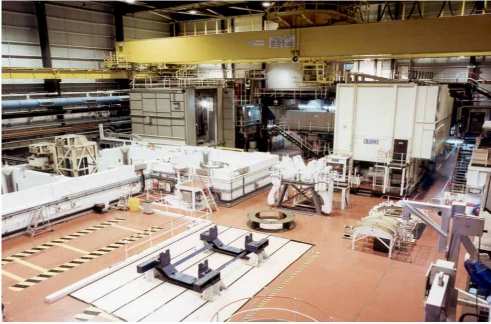
Fig 6 Oxide Flask Maintenance Facility
