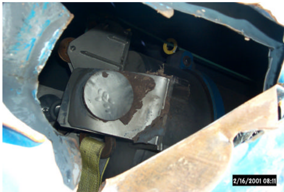
View into IP-2 Showing Damage to Transfer Cask Operator
