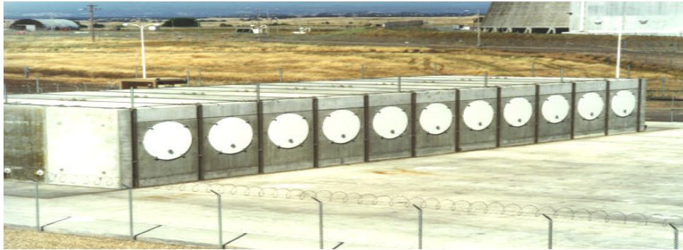
Array of NUHOMS® Storage Modules
