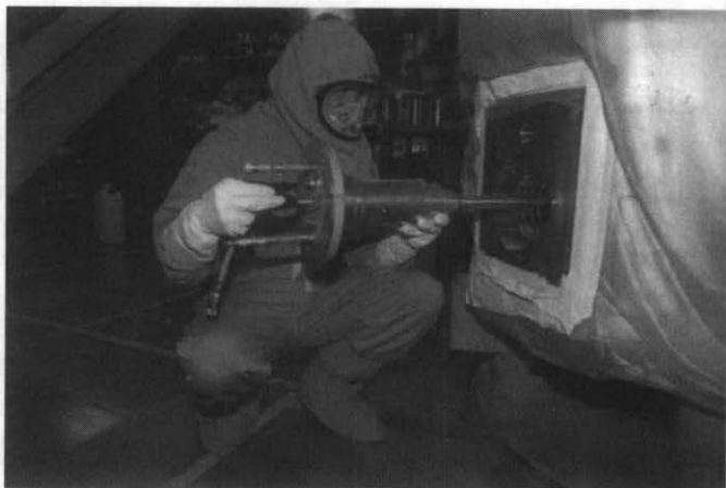
Insertion of a counter-electrode into one of the lower orifices
