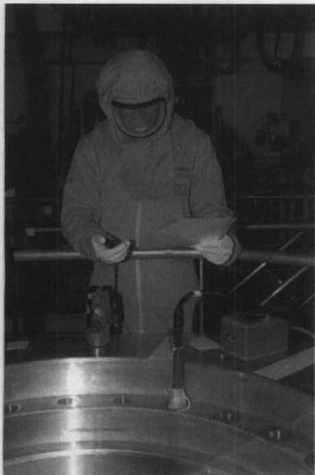
Treatment of plug flat walls using a mobile buffer
