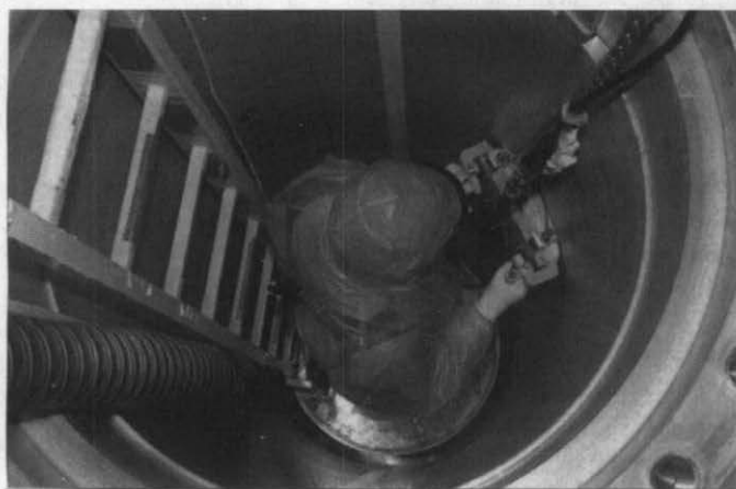
Treatment of cavity interior using a mobile buffer
