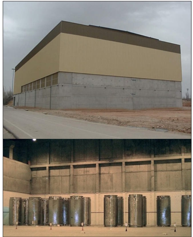
Figure 6. Trillo ISFSI and ENSA-DPT casks inside the building
