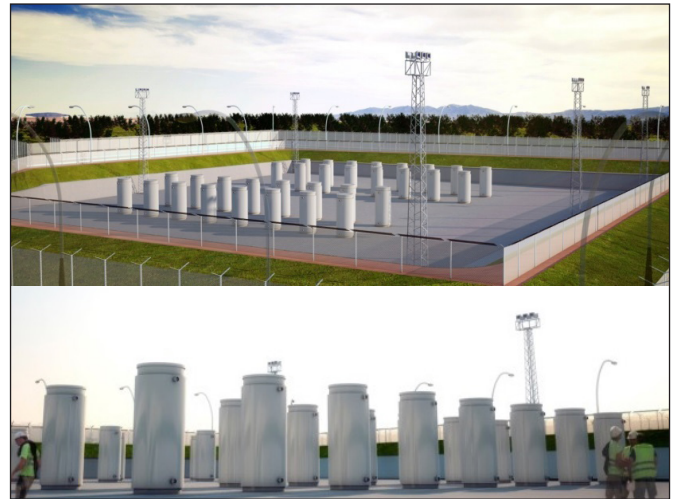
Figure 11. Santa María de Garoña ISFSI and ENUN 52B in the concrete pad (artist views)
