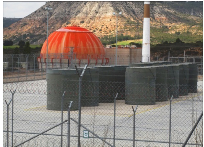
Figure 8. José Cabrera ISFSI and HI-STORM 100Z in the concrete pad
