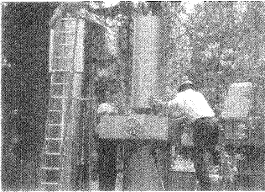
The facility transfer shield, loaded with spent fuel, is transferred out of the reactor building for loading in the transfer cask and NAC-LWT.
