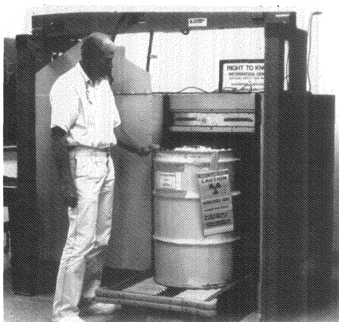
Figure 9. Photograph of the waste drum assay system.
