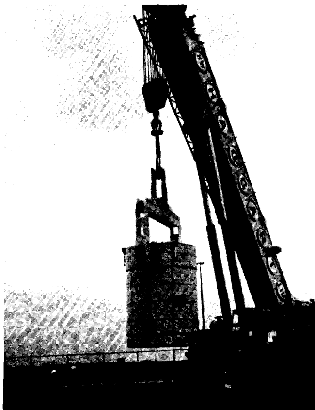
Figure 9. Placing the loaded CIC on the timber crib for storage
