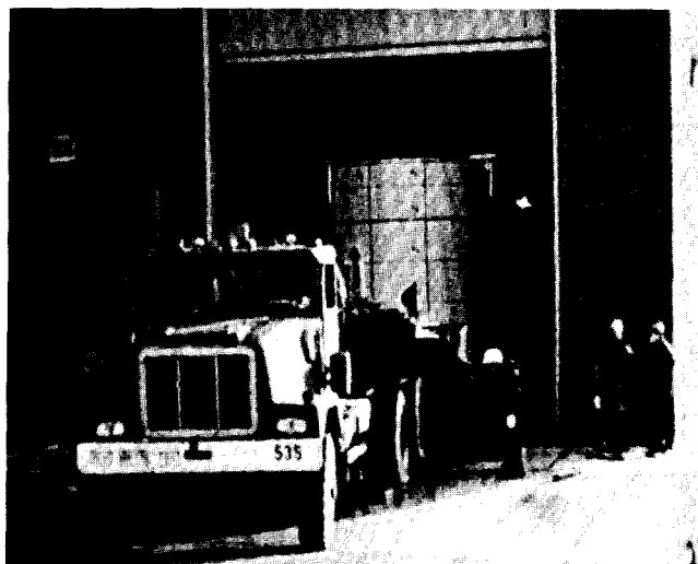
Figure 4. Transport of CIC to reactor building
